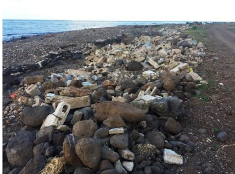
Concrete debris used for sea protection
